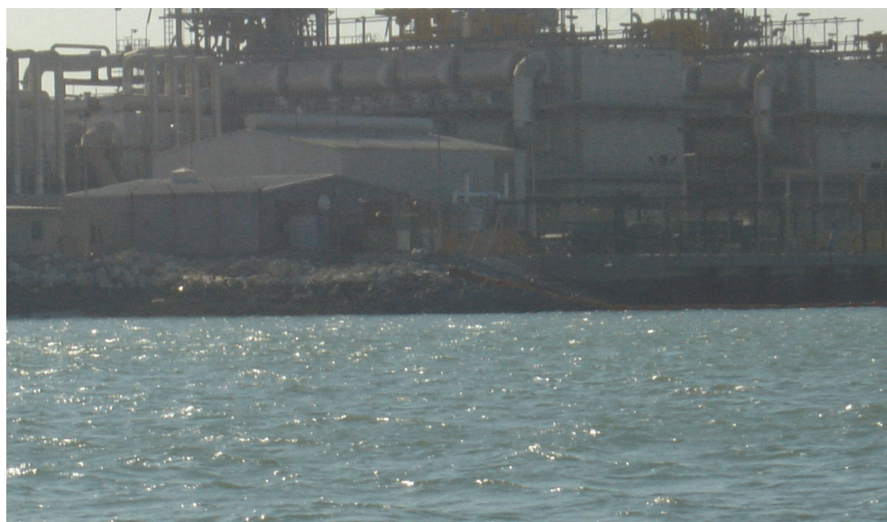
Fig. 4. Sitra Power and Water Station.
