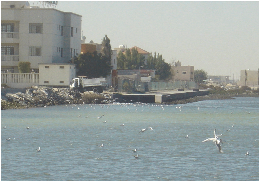
Fig. 3. The outfall of Tubli Water Pollution Control Centre, the main sewage treatment plant in Bahrain.
